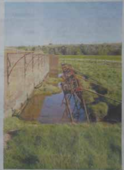
GREAT SURVIVOR The remains of a First World War rifle range near Humphrey Head, Kents Bank. The pond at the base is now a home for minnows
