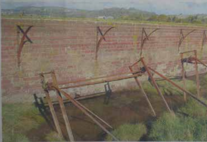
TAKE AIM Part of a rare First World War rifle range near Humphrey Head, Kents Bank. Targets would be moved into position using pulleys
